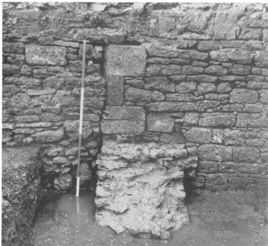
Plate 44. Greyfriars, Site B. Phase IV. The S. corner of the W. wall of the N. nave, B X F1 (right), resting on the foundation of the Phase II N. wall of the N. aisle, B X F2, before dismantling. The Phase VIII blocking wall, B X F4, is to the left with the post-medieval property wall superimposed across the top of both walls. View from the E. Scale 2 m. Photo by K.W. Sheridan.
