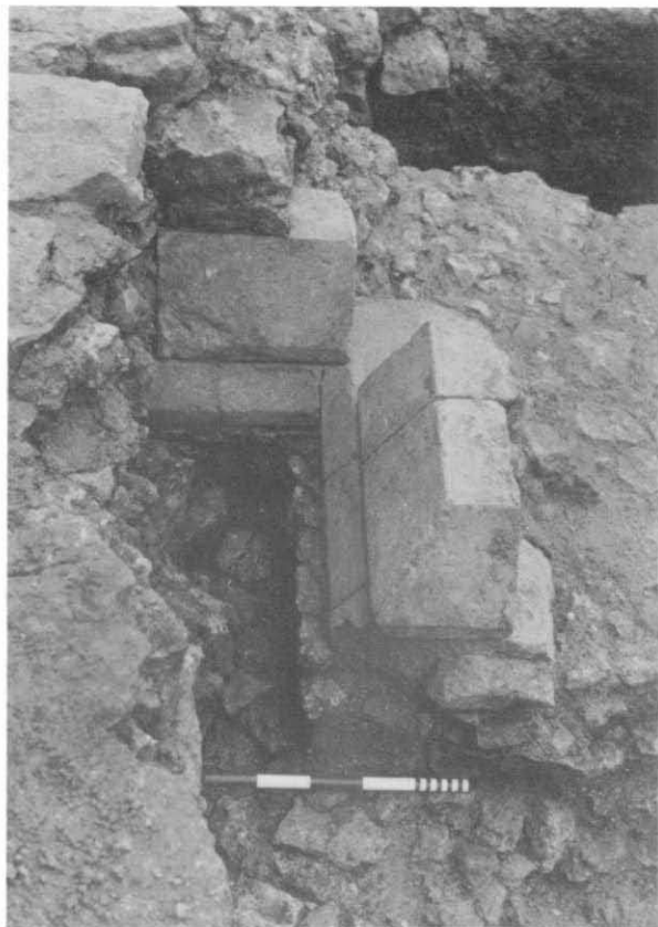
Plate 41. Greyfriars, Site B. Phase II. The eastern plinth (Worked Stone Cat. No. 2) of the buttress B X F2, after the removal of the W. wall, B X F1, of the N. nave. View from the N. Scale 0.50 m. Photo by K.W. Sheridan.
