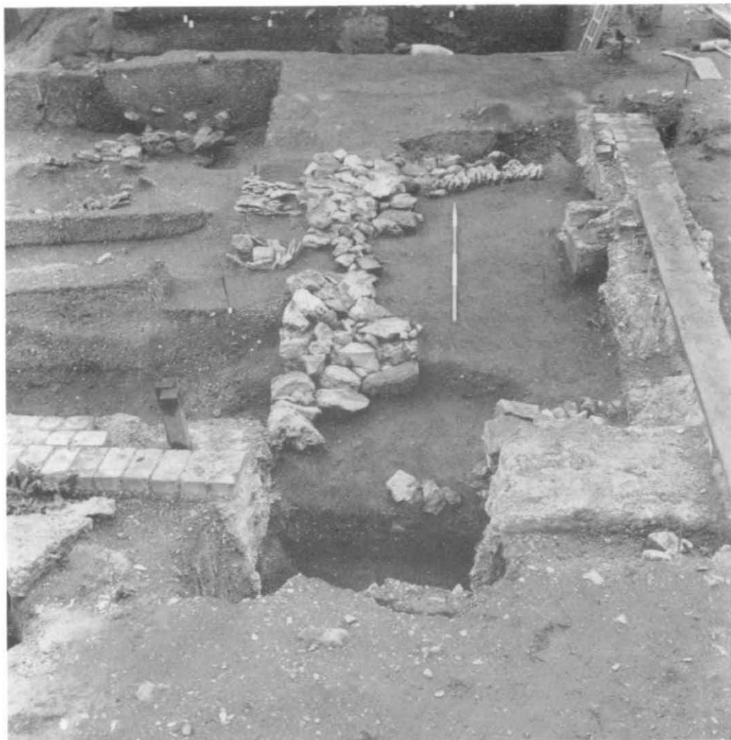
Plate 13. 31-34 Church Street, Site A. Rear wall of No. 31 (SW82). Whitehall A F8. View from the W. Scale 2 m. Photo by K.W. Sheridan.
