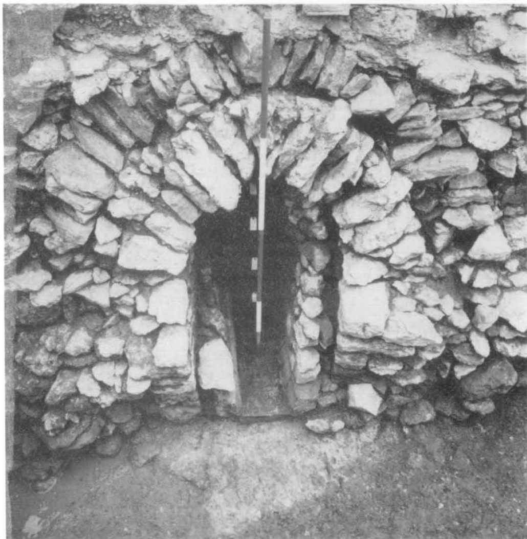
Plate 36. Greyfriars, Site B. Phase I. The N. side of the culvert in the N. wall of the choir, B I F2. Scale 2 m. Photo by K.W. Sheridan.
